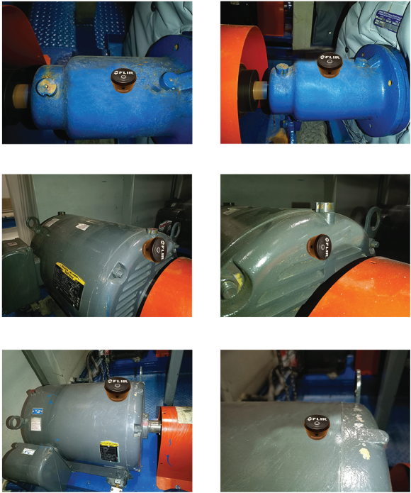
Figure 10.2 Sensors shown mounted on machinery.
