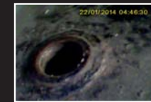
Inspection bore of tank using 6mm Long Focus camera (VSA2-1)
