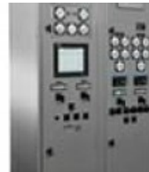
Zenith Energy Commander* Paralleling Switchgear (PSG)
